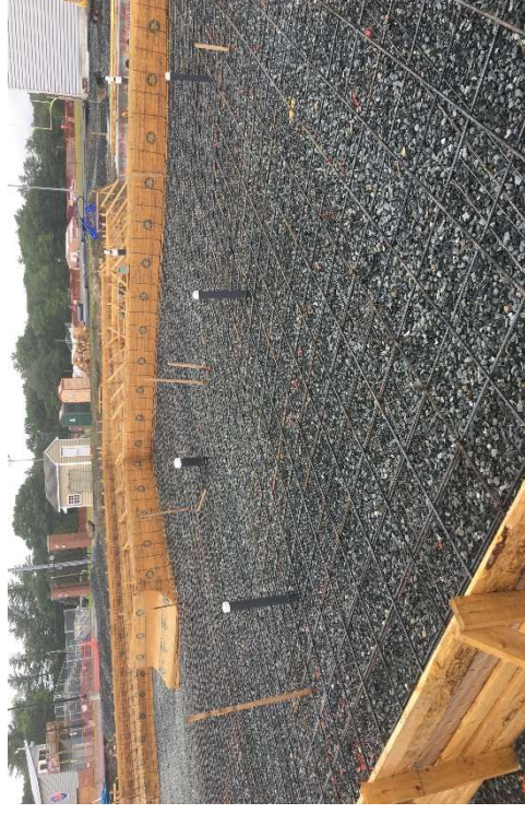
Formation of Pool Shell and Steel Work
