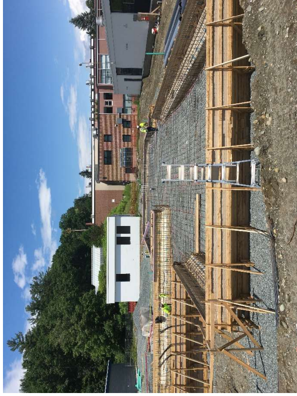
Formation of Pool Shell and Steel Work
