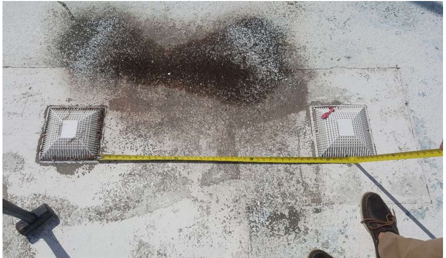
Figure P: Wading Pool Main Drains
