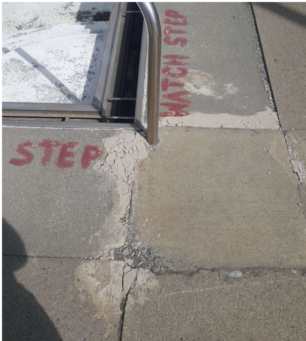
Figure G: Settled/Cracked Deck
