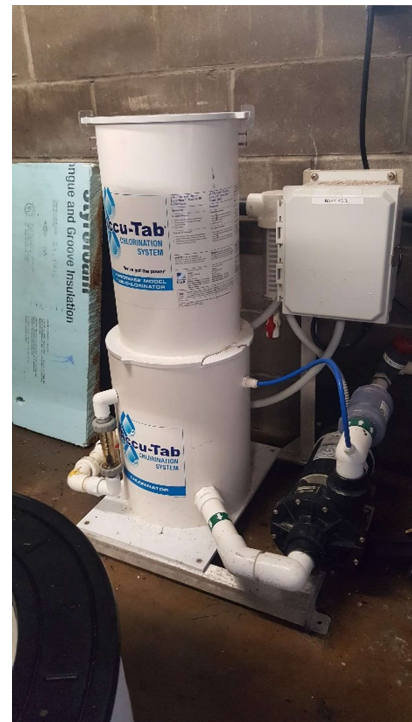
Figure U: Tablet Feeder
