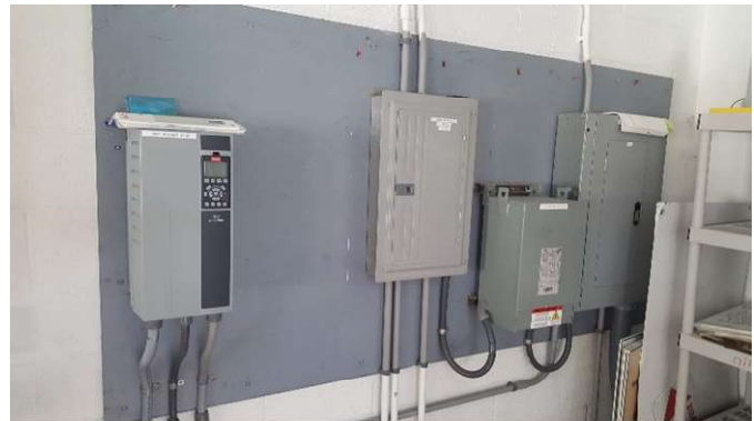
Figure V: Electrical Panels and Motor Starters
