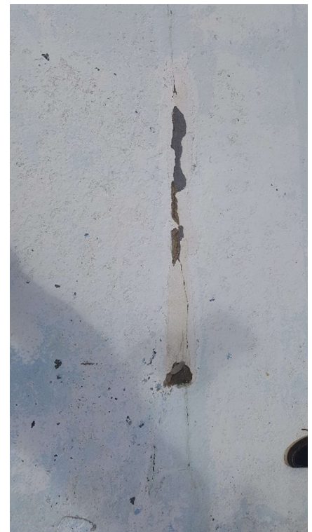
Figure J: Pool Wall Cracking
