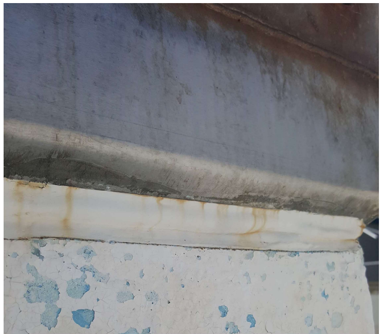
Figure D: Current Gutter/Wall Expansion Joint
