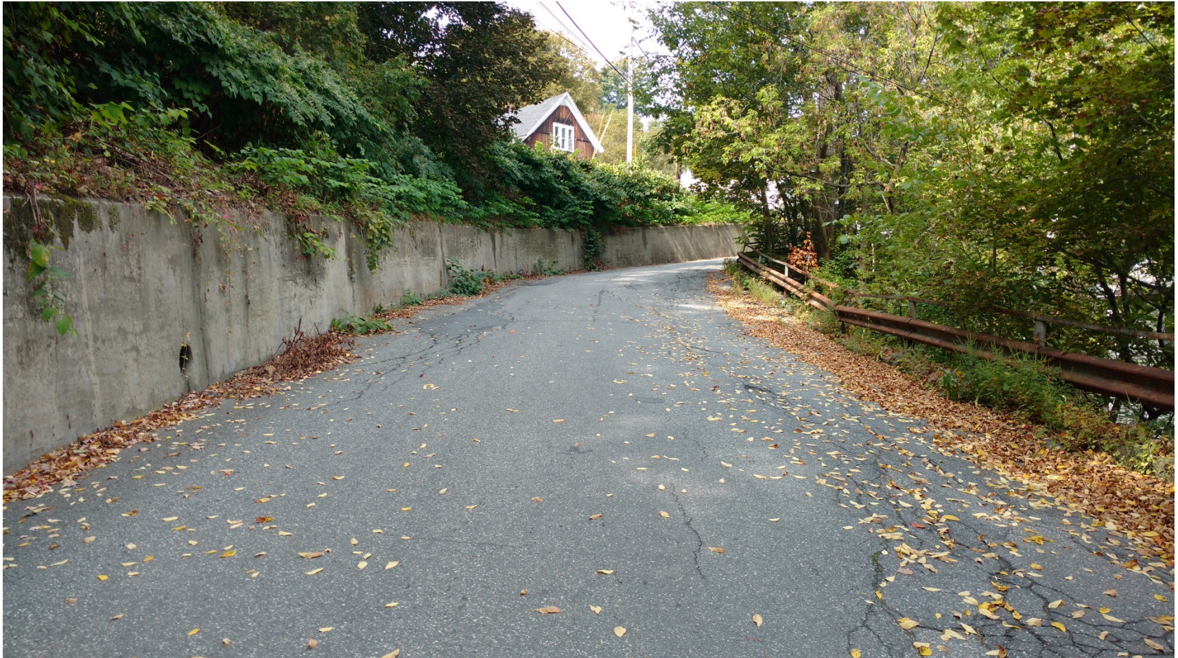
Segment 1B: Poor Condition w/non compliant guardrail (over the bank on the right hand side)
