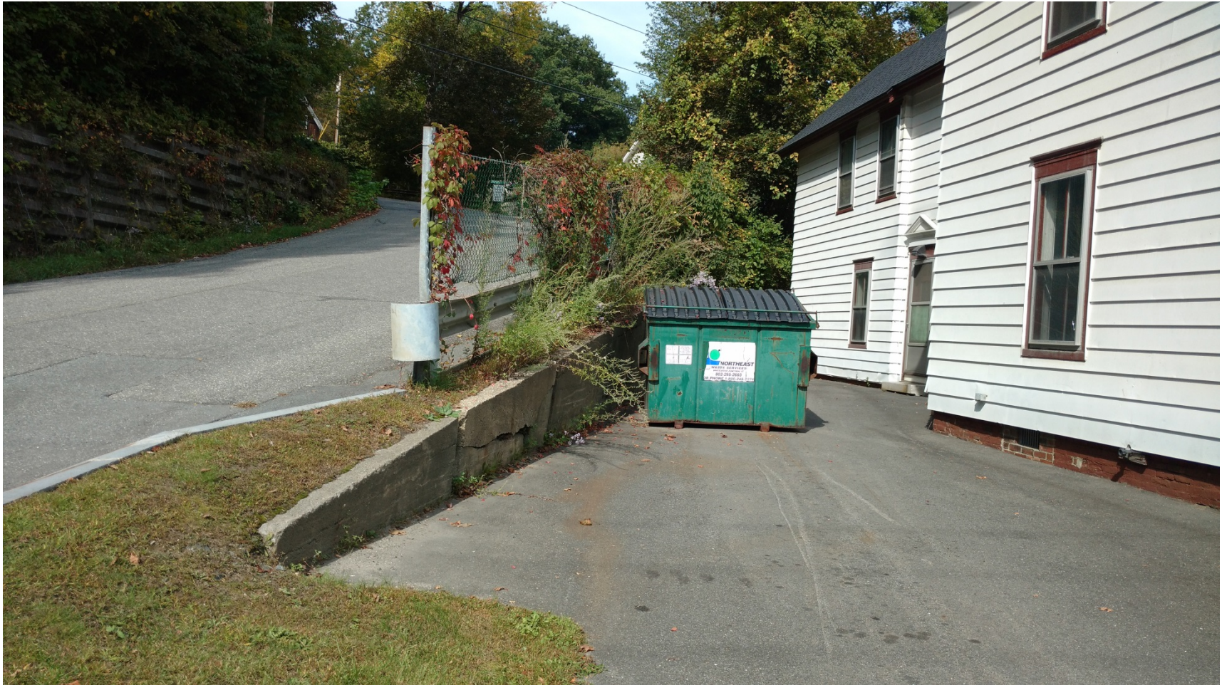
Segment 2: Concrete Wall (fair condition with AOT compliant guardrail)
