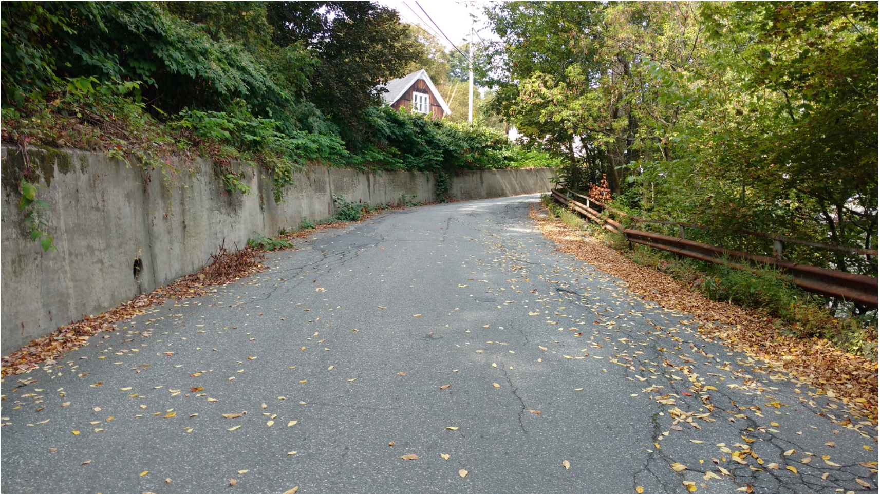
Segment 4: Concrete wall on the left (good condition, slight deficiency in sliding)
