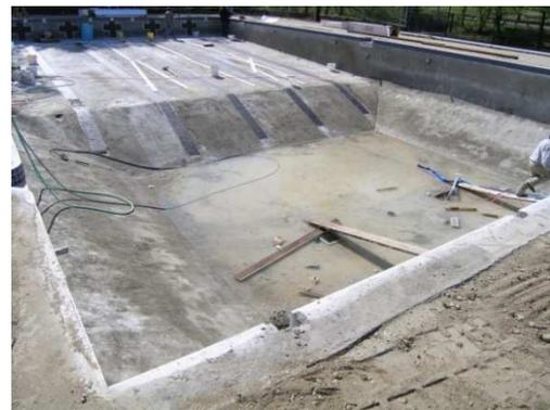
*Pool-In-Pool Construction to Repair Tank and Shallow Deep End, saves on demolition, dewatering and foundation costs*
