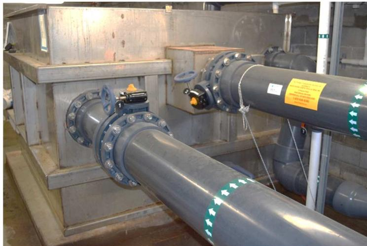
*The existing stainless DE filter can be incorporated as a surge tank or backwash storage tank saving the cost of removal.*
