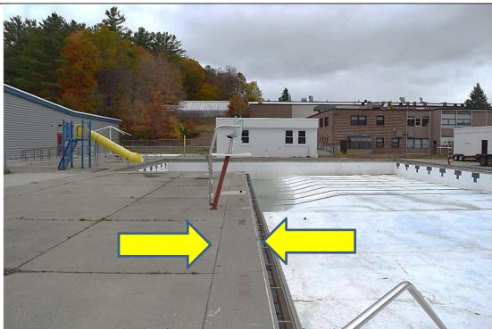
Area of Deck Replaced when gutter was installed in 1997
